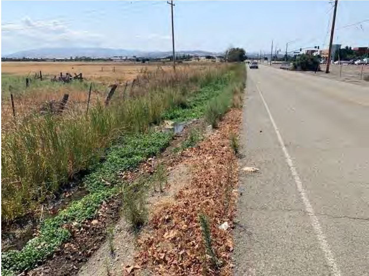
PHOTO 1.2-2: Typical conditions of Jordan Creek (roadside channel) adjacent to existing Fallon Road downstream of the Dublin Boulevard alignment. Little sinuosity in low-flow channel and narrow overall cross section.
